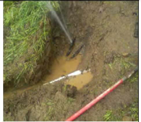
Leak repair in our system.
