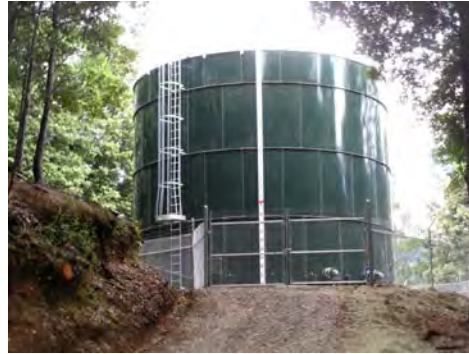
New Bussell water tank Completed June 2016
