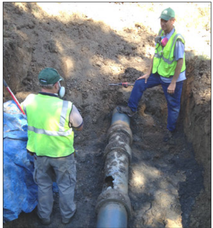
~10 inch main line water leak! ~
