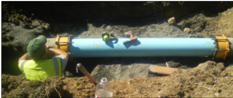
~10 inch main line repaired! ~
