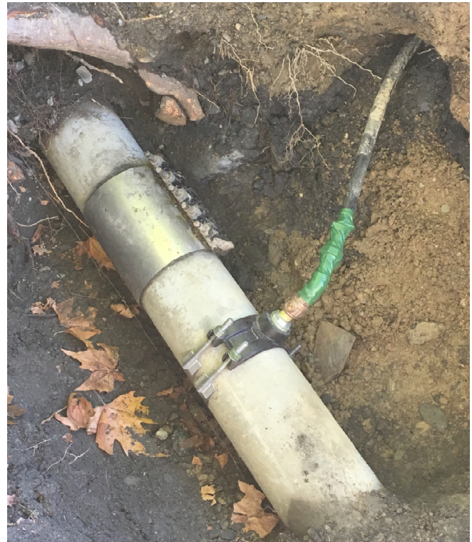
~Repair clamp and new service saddle~
