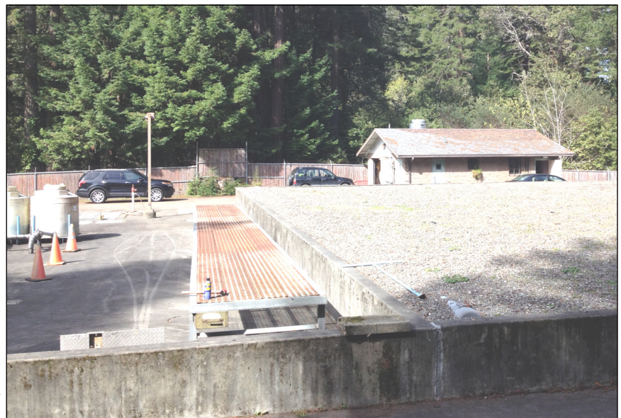
~Wastewater Treatment Plant similar to what Willow Creek will have~
